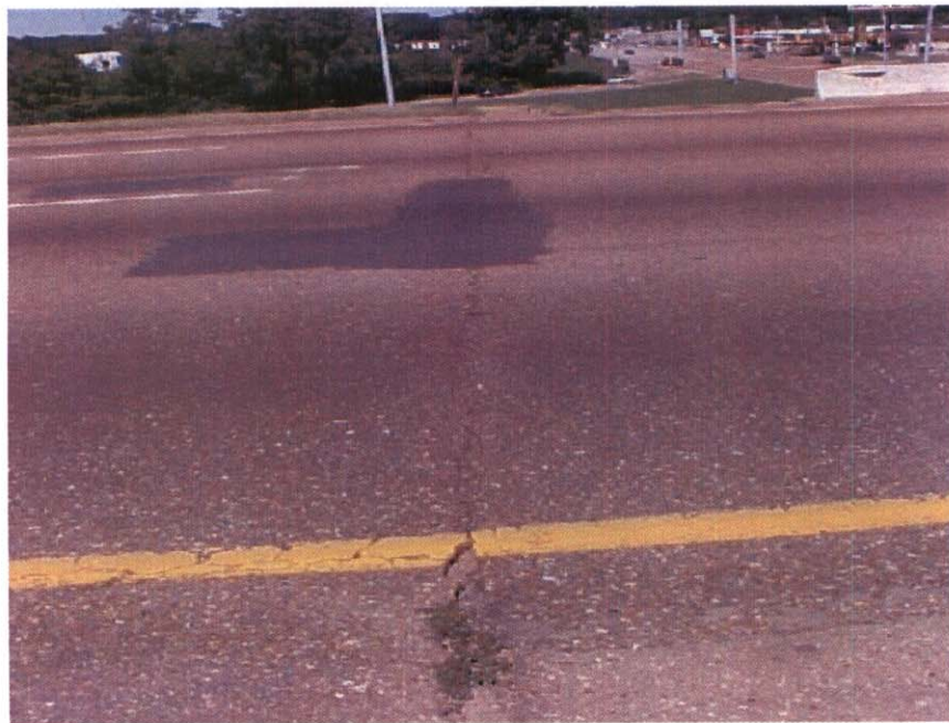
APPROACH #1 PAVEMENT CRACKING & SPALLING
