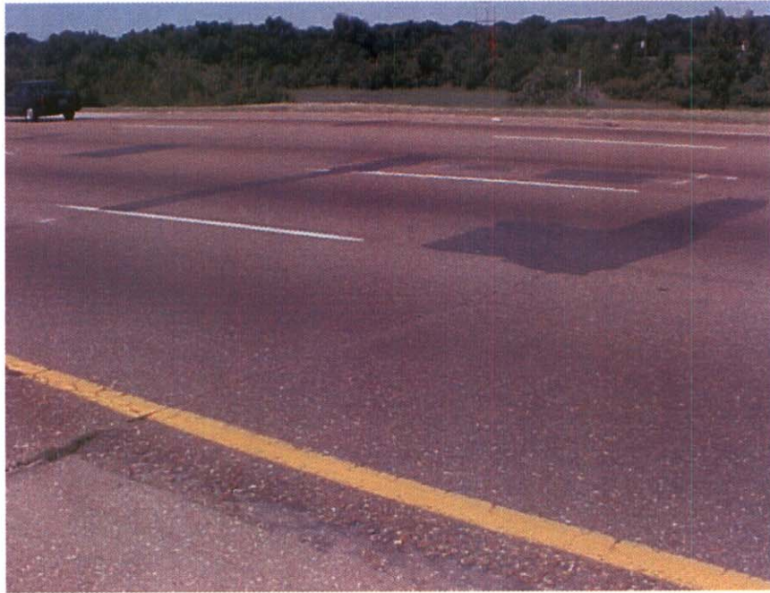
APPROACH #1 PAVEMENT CRACKING & SPALLING
