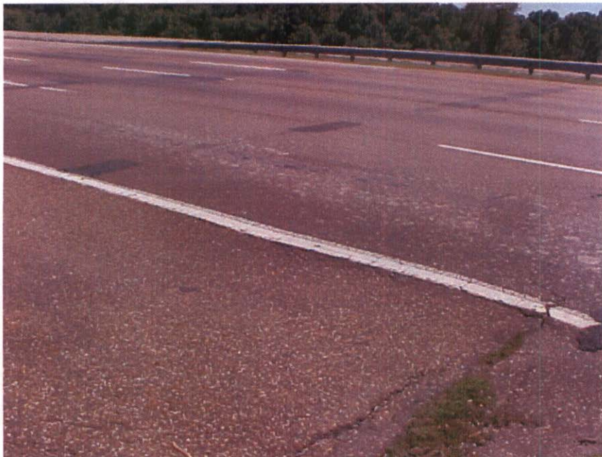
APPROACH #2 PAVEMENT CRACKING & SPALLING
