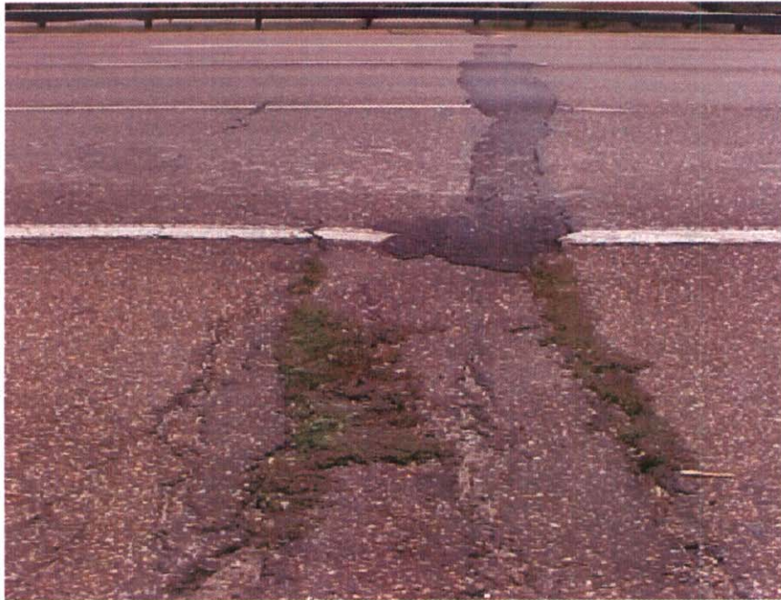
APPROACH #2 PAVEMENT CRACKING & SPALLING
